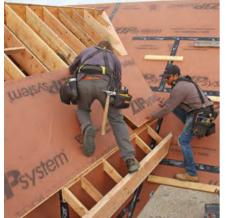
WORK TOWARD THE VALLEY With the first piece of sheathing in place, I measure to the valley from the top and bottom of the first panel to determine the angle on all of the sheathing panels that abut the valley. I transfer those measurements to the panel, cut it, and nail it in place.
