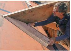
**SCRIBE THE TOP** I find the angle of the valley plate by scribing it on a scrap and then measuring the angle with a speed square. Then I check the fit for accuracy. A 33° bevel on the plate provides solid attachment for the roof sheathing installed later.
