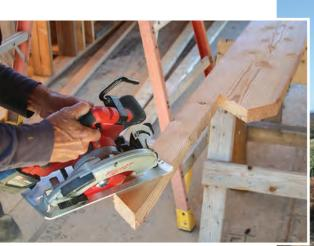
TRIM THE END Common rafters that butt into the main roof need their tails trimmed. I cut the rafter tail with a compound cut to match the slope of the main roof. I leave 1½ in. between the end of the rafter tail and the main roof to leave room for roofing and flashing.
