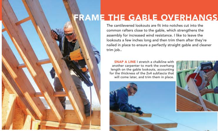
NAIL THE LOOKOUTS We drive screws through the tops of the 2x4 lookouts and into the rafters at the notches, and then through-nail the ends of the lookouts where they meet the rafter.
