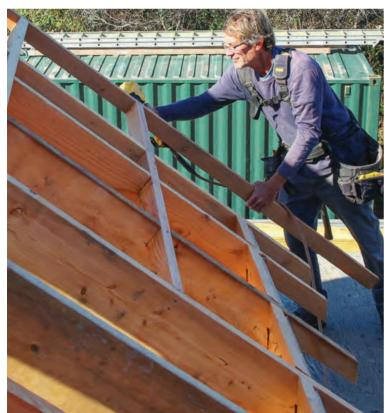
FASTEN THE RAKE SUBFASCIA... I cut the subfascia from a single 2x4 free of splits or large knots to make the overhang stronger. I also make sure it's straight, which makes installing the finished 1x trim and beadboard on the overhangs easier and ends up looking better.
