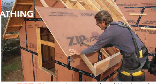
**START STRAIGHT** I measure up from the overhang and snap a chalkline to line up the first course of panel roof sheathing, which starts at the plane of the exterior wall. I nail the sheathing with 2½-in. galvanized ring-shank nails every 4 in. on panel edges and 6 in. on center in the field.
