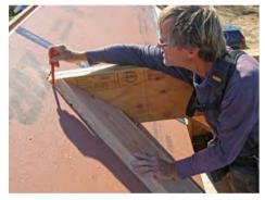
MARK THE POSITION Once I've dialed in the angle, I hold the scrap so the top edge aligns with the top of the ridge, and then mark the end of the plate on the ridge.
