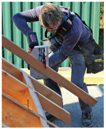
...AND TRIM IT IN PLACE Once the subfascia is nailed in place, I cut the excess with a circular saw. To mark the cut, I extend the overhang length from the rafter tails using a chalkline aligned with the rafter tails that are already trimmed.
