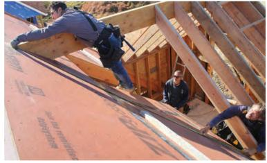
**MEASURE** THE PLATE To determine the length of the valley plate, I stretch a tape measure from the mark I made on the ridge showing the end of the valley plate down to the center of the valley. This will be the longer side of the plate.
