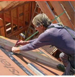
LAY OUT THE JACK RAFTERS I measure from the common rafters to continue the rafter spacing on the valley plate. The rafter spacing can also be determined with a rafter square or construction app or calculator, but on a small roof like this I find measuring in place is faster.
