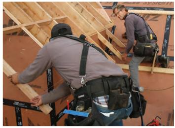
MARK THE LENGTH OF THE OVERHANG Holding the tape measure level, I measure from the edge of the wall sheathing to mark and trim the overhang. The 12-in. overhang will have a 1½-in.-thick subfascia, so I mark both ends of the overhang at 10½ in. and then snap a line between the marks to indicate where to cut the rafter tails and rake subfascia.
