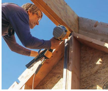
**LEVEL AND NAIL THE RIDGE** One end of the 2-ply LVL ridge is cut at a 40° angle to match the 10:12 pitch and bears on the header in the main roof. The other end fits into a beam pocket above a post on the gable end.
