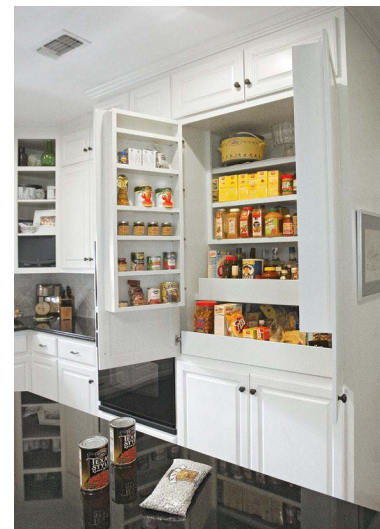
Pantry in place. When there's no space outside of the kitchen for a pantry, put it in the kitchen. This pantry cabinet has storage behind the doors, on lower pullout shelves, and on shelving on the back side of the doors.
