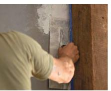
Finish to finish. It's easier to mold wet plaster to solid trim than it is to scribe solid trim to rock-hard plaster, so install trim before plastering. Rabbet the backside of large wood trim and tuck plaster behind it to prevent gapping as the trim expands and contracts.
