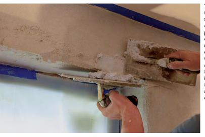
Two-trowel technique. Use two trowels—one to apply plaster, and one to hold material and catch drops—when working areas where the plaster has a harder time sticking, such as outside corners.
