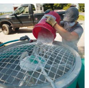
Master the mix. For this process, the ratio of hydrated lime to sand should generally be at least 1:2, but no less than 1:4. Wear a suitable respirator when mixing to avoid breathing in the lime.
