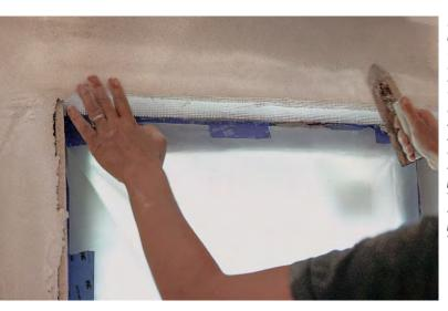
Fiber reinforcement. Reinforce inside and outside corners with drywall mesh tape to add strength and prevent cracking. Apply a layer of plaster, embed the tape, and apply more plaster to bury the tape.
