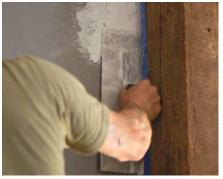
Smooth it out. Use a pool trowel to smooth the plaster without leaving tool marks behind. For added texture, smooth with a square-edged trowel first, then a pool trowel after the plaster has firmed up a bit.
