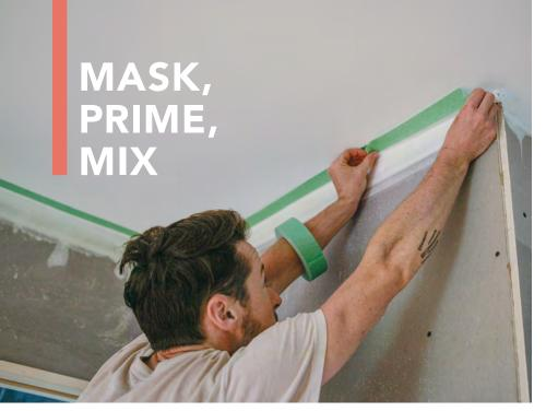
**Screed to tape.** Use painter's tape to establish the thickness of the plaster, setting it to ½ in. to ½ in. out from the wall on all of the trim, ceilings, and windows. The tape serves as rudimentary screed lines, and it protects adjacent surfaces from the mess of plastering.
