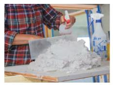
Plasterer's setup. Set mortar boards at a comfortable height, and temper the plaster with spritzes of water as needed to maintain its consistency. Dedicate a worker to refilling mortar boards so the plasterers can focus on plastering.
