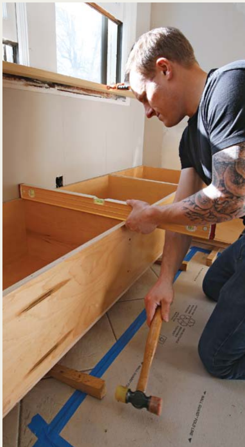
Wedges before shims. Reusable oak wedges are larger and steeper than typical shims, making them ideal for quickly and temporarily getting carcasses into position before shims are added.
