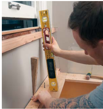
Accurate angles. Adjust the bottom nailer in or out at each screw location until a digital level reads 83°—a perfect 7° slope—before fastening the nailer to the lid cleat below.
