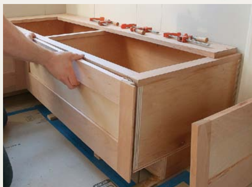
Skin the boxes. Trim each front panel to length, and fasten it to the carcass face with finish nails.
