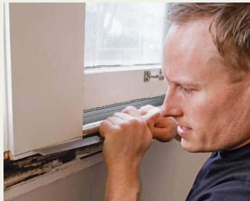
Make way for the cap. If tying the bench seat into a windowsill, strike a level line across the window casing. Cut along the line with a handsaw or multitool, and remove the molding.
