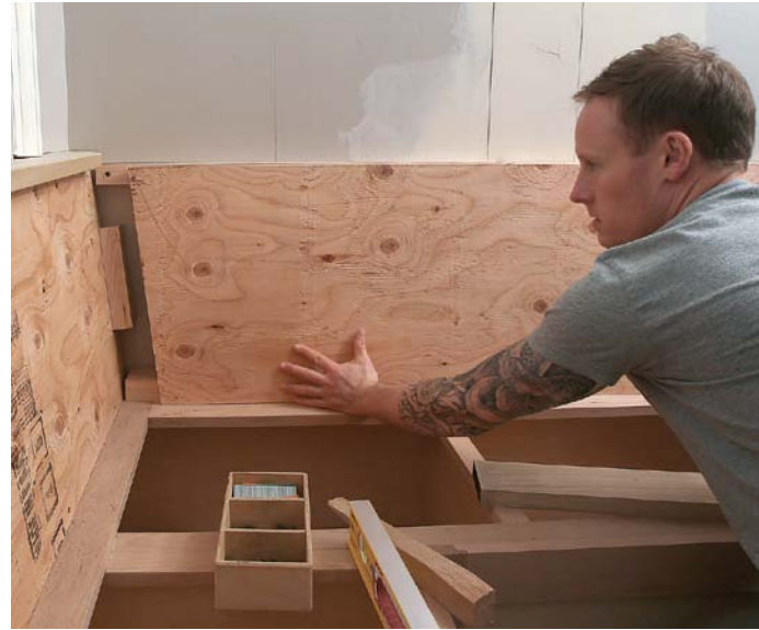
Beveled backrest. To create a sturdy backrest subbase, fasten \frac{3}{4} -in. CDX plywood with top and bottom bevels to the upper and lower nailers.
