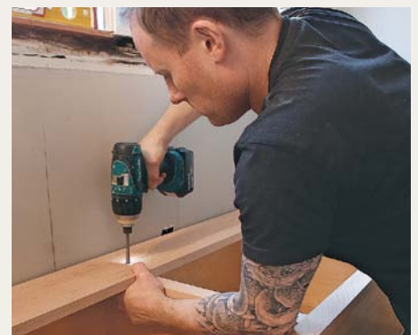
Lid cleat does heavy lifting. This 1x6, referenced off the front edge of the carcass, supports the backrest assembly and the lid hinges.
