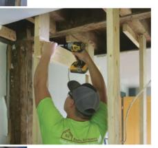
walls can be useful too. If you screw a strut between them, you can catch the beam that is coming out or help support the new beam when it is being raised.
