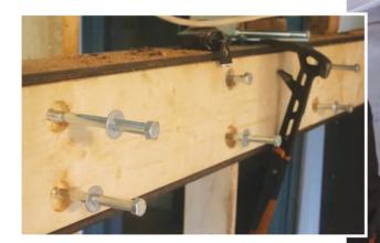
are usually specified by height and weight per foot. The two beams we used are W8x28, which specifies a wide-flange I-beam that is 8 in. tall and weighs 28 lb. per linear foot.
