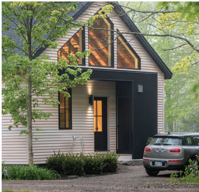
REVISED EDITION From a distance, the clapboard siding mimics the original barn's siding to stay in keeping with the neighborhood. Existing windows were replaced with Marvin Elevate triple-pane units—chosen for their minimal trim—which required installing window bucks. There are new patio doors on the east that replaced an old sliding barn door and modern gabled glass on the west.
